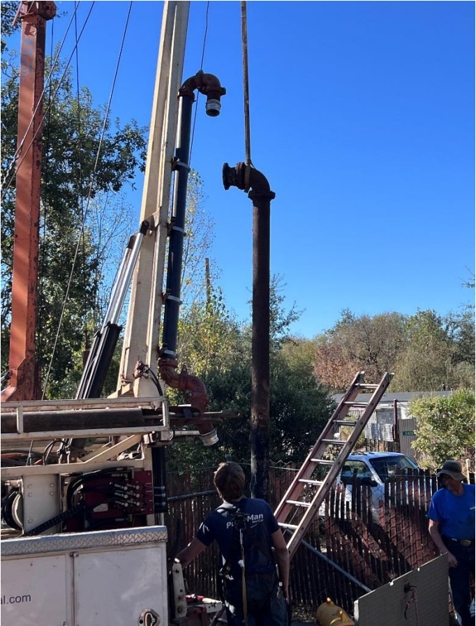
PumpMan removing a section of ductile pipe from the wet well.
