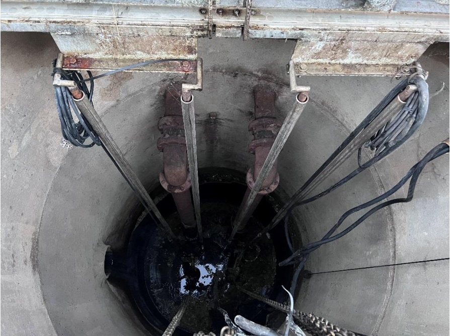
Original piping and slide rail system to be replaced.
