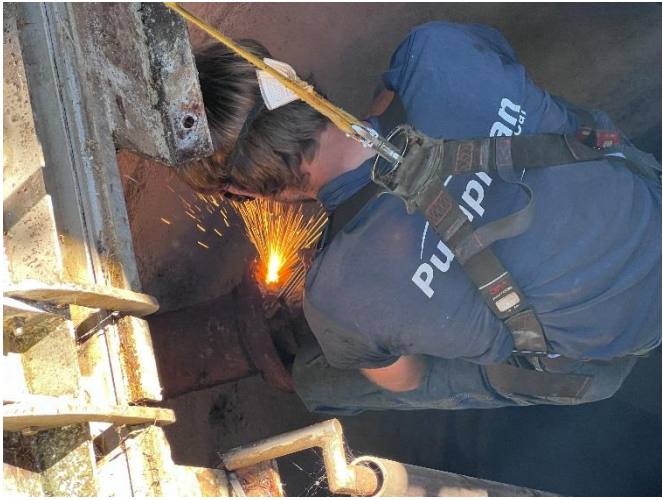
PumpMan removing a section of ductile pipe from the wet well.
